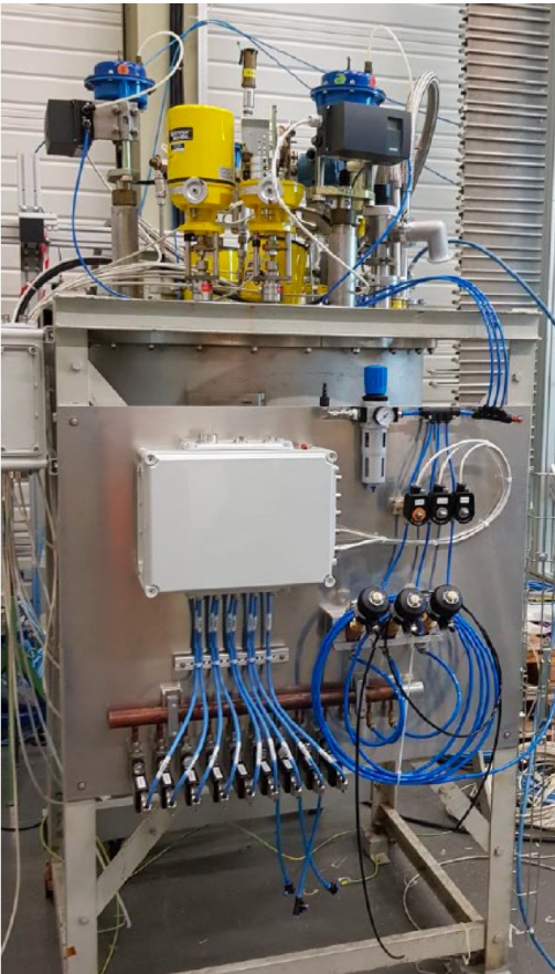
new LN 2 cooling system control for Si (EP-DT)
