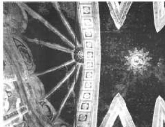
Figures 2 & 3: (left) the frescoed apse before the restoration, damage is diffused at the basis of the wall and (right) the vault before the restoration, the fresco has stains due to many infiltrations
