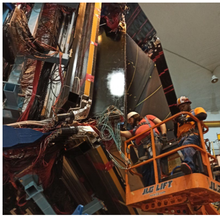
(a) Cabling the RICH
